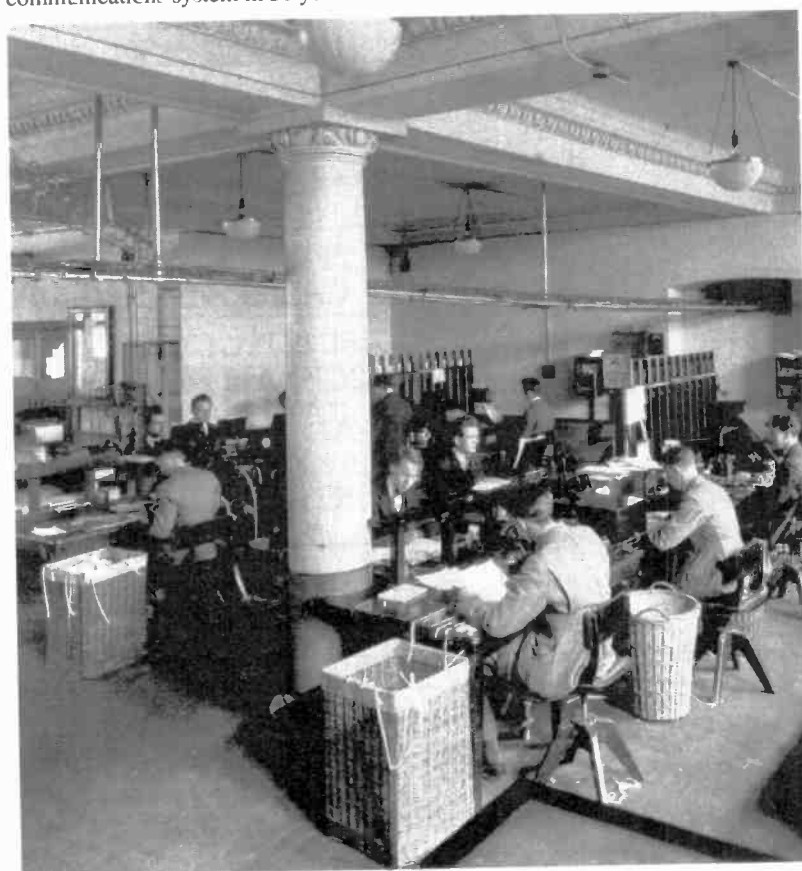
Central Telegraph Office at Radio House.
