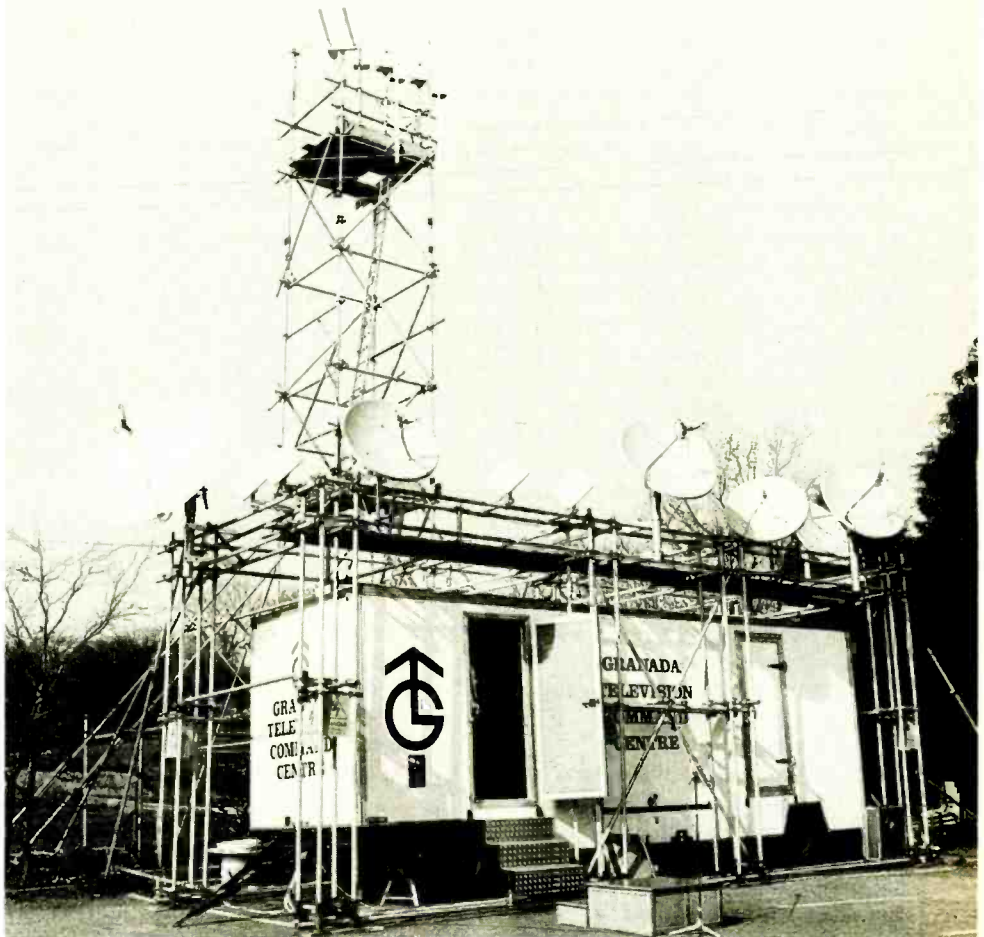
Command centre for the village channel was a Granada trailer surrounded by scaffolding to support aerials and with a tall tower for the MVDS transmitter.
