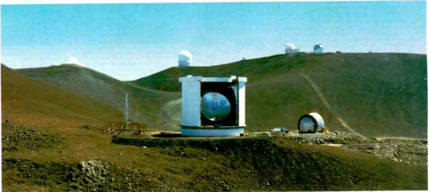
The James Clerk Maxwell Telescope, the Mauna Kea. The viewing aperture can be covered by a p.t.f.e. membrane.
