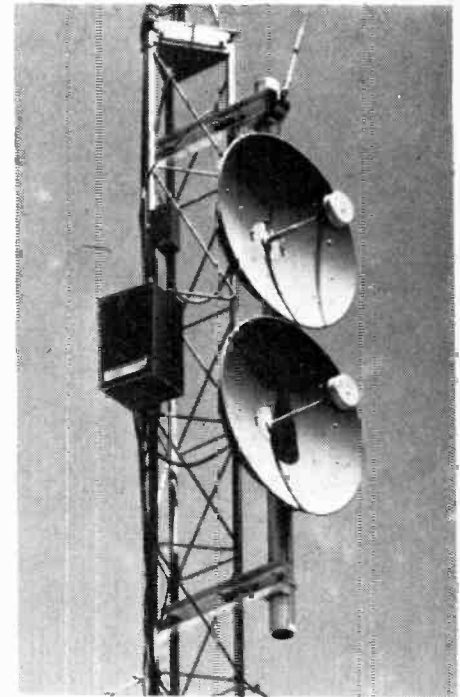
Fig. 6. A receiving location aerial tower. The lower dish is used for TV pick-up and is connected to the down-converter bolted to the tower. The upper dish is used for the audio talk-back transmission.
