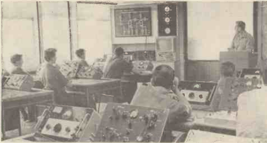
A technicians' class receiving instruction with the aid of a demonstration console, on which a wide variety of circuits with plug-in assemblies or components can be used.
