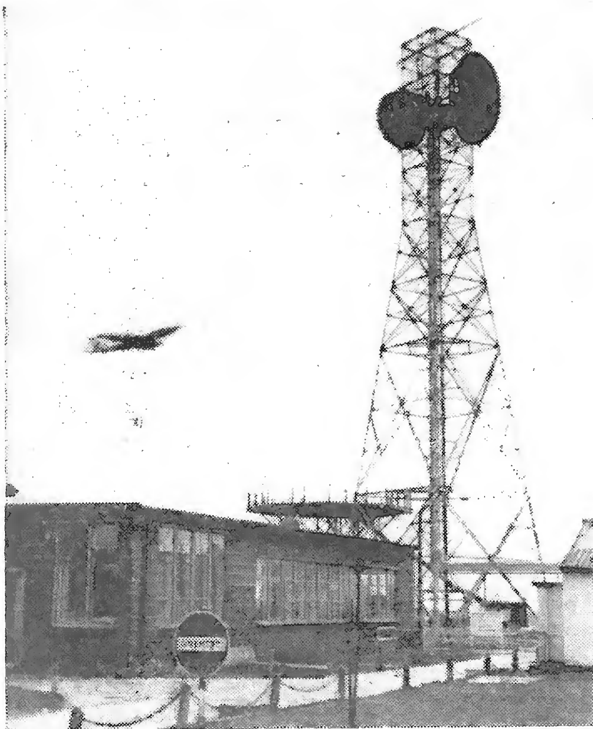
The three dishes on the tower at the S.A.T.C.C., near London Airport, receive via microwave links radar information from sites at Ash, near Dover, Ventnor, I.o.W., and Clee Hill, Shropshire.
