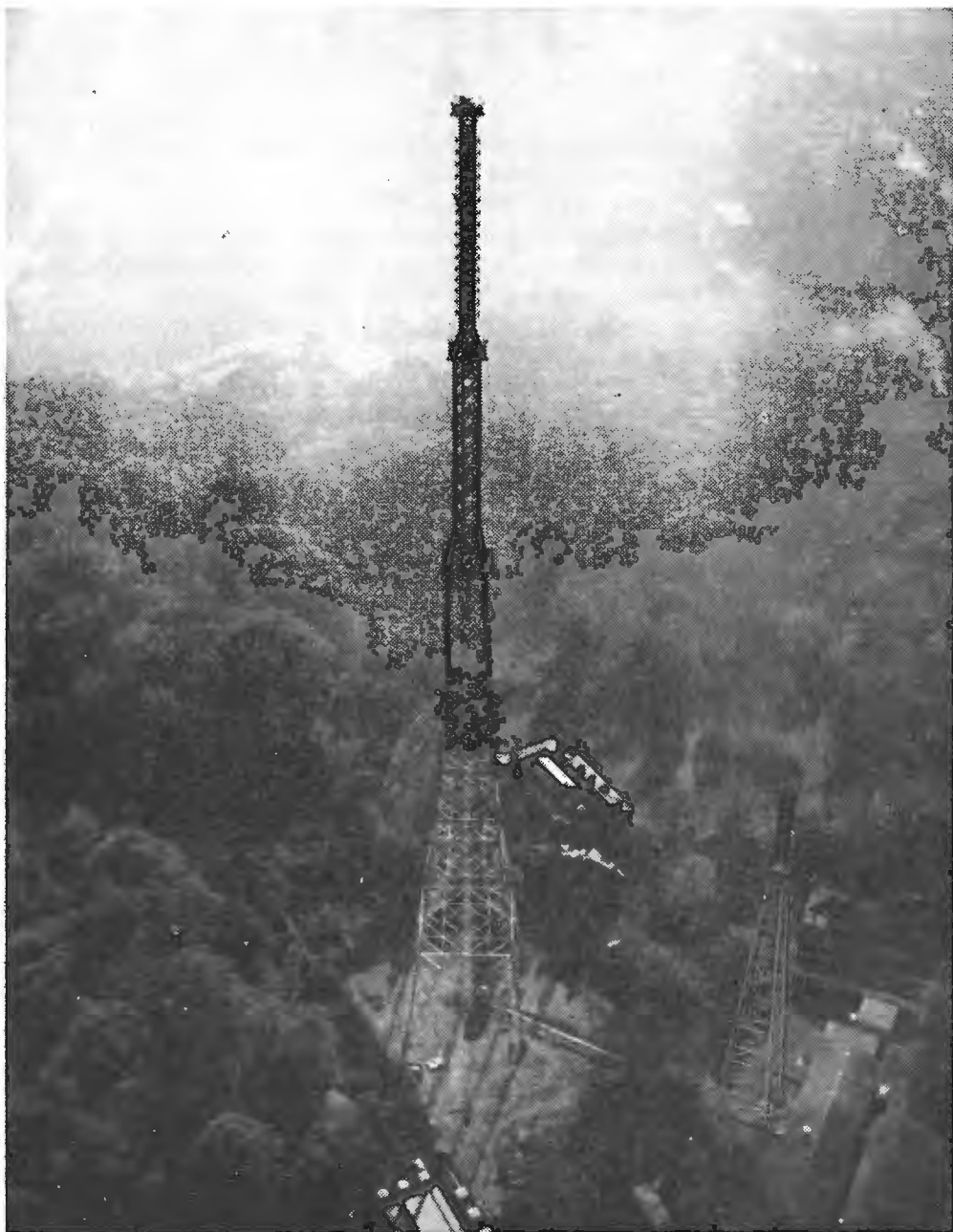
This aerial photograph (by Barnet Saidman, F.I.B.P., F.R.P.S.) emphasizes the slim design of the new 500-ft. I.T.A. television tower at Beulah Hill, Croydon, and incidentally the small area of the available site. The old 200-ft. aerial is just discernible to the right of the new tower.
