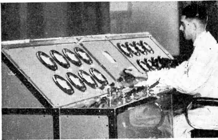
(Left) Marconi-E.M.I. "instantaneous" camera, so-called because the Baird system employed intermediate film scanning. The cameraman is D. C. Birkinshaw, now Superintendent Engineer, Television.
