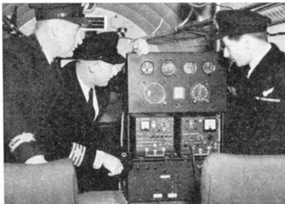
Doppler navigation equipment (Marconi) in a Viking aircraft.
