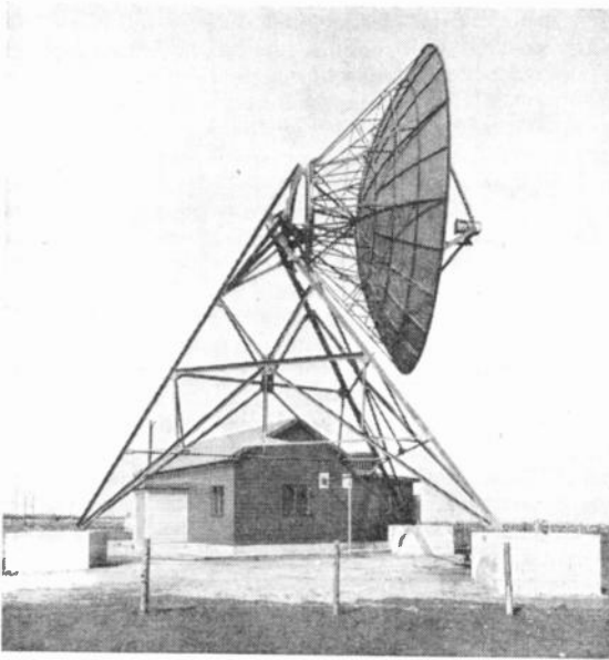
Experimental tropospheric scatter station at Start Point: frequency 858Mc/s, power 10kW.
