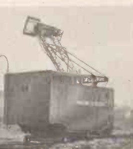
EXPERIMENTAL tropospheric scatter transmitter installed by Marconi's at Great Bromley, Essex. The 30-ft reflector is energized by a horn mounted on the transmitter vehicle which is moved on an arc of railway track to "steer" the transmitted beam. The working frequency is 858 Mc/s.
