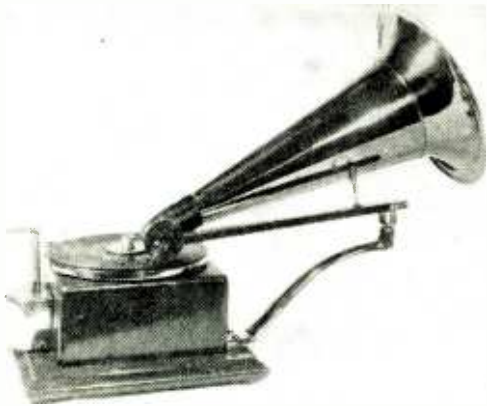
1897 needle-using disc gramophone
