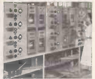
Testing—Grid Current Recording
