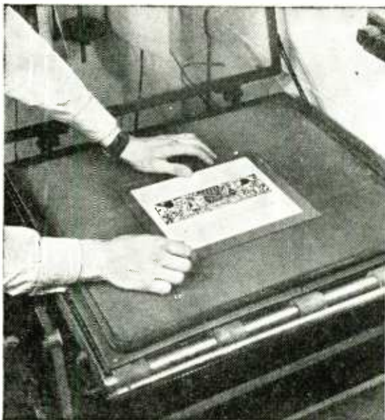
Preparation of the silk-screen master from the photographic plate.
