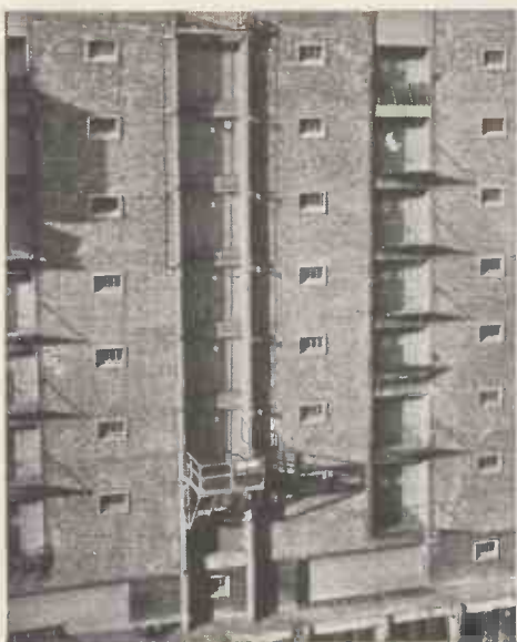
An electrically operated rising platform in use at Butler's Wharf Ltd., London. It can be quickly locked into position at any floor, and is a great time saver.
