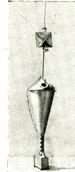
The Venner wireless transmitting buoy is designed to minimize rolling and weighs only 300 lb.
