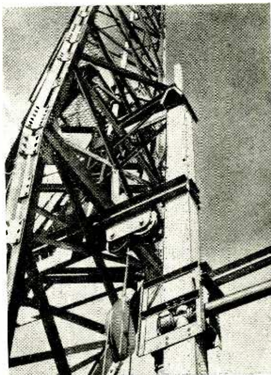
View from the bottom of the mast at Kirk O'Shotts, showing how the feeder is led in. The pulleys are part of the loading mechanism.
