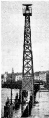
The scanner of the Douglas Harbour radar installation on its 60-ft tower.
