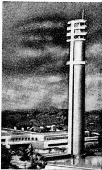
MICRO-WAVE TOWER. A reproduction of the architect's model of the Federal Telecommunications Laboratories, New Jersey, showing the 300-foot tower which will be used for U.H.F. research.
