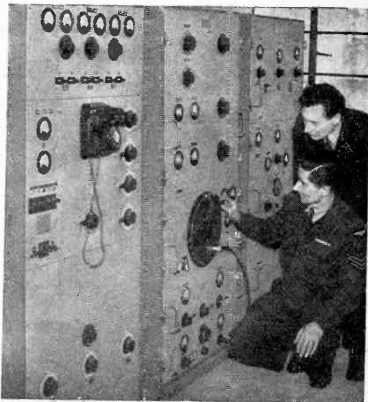
The centre unit is the transmitter — a Rediffusion G12 (R.A.F. Type J 1412)—with (left) the control unit and (right) the power rack. The lower photograph shows the insulated base of one of the three 300-ft vertical radiators which are arranged in line about two miles apart.
