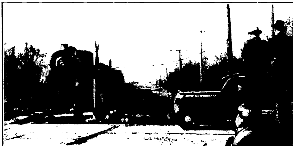
WHAT NEXT! To avoid the many fatal accidents that are caused by collisions at level crossings between cars and trains, an American engineer has devised a signalling system, actuated by rail contacts, whereby the driver of a car fitted with a receiver embodying the necessary device is given warning of the approach of a train. The transmitter giving the warning signal is stated to have a range of 1/4 mile.
