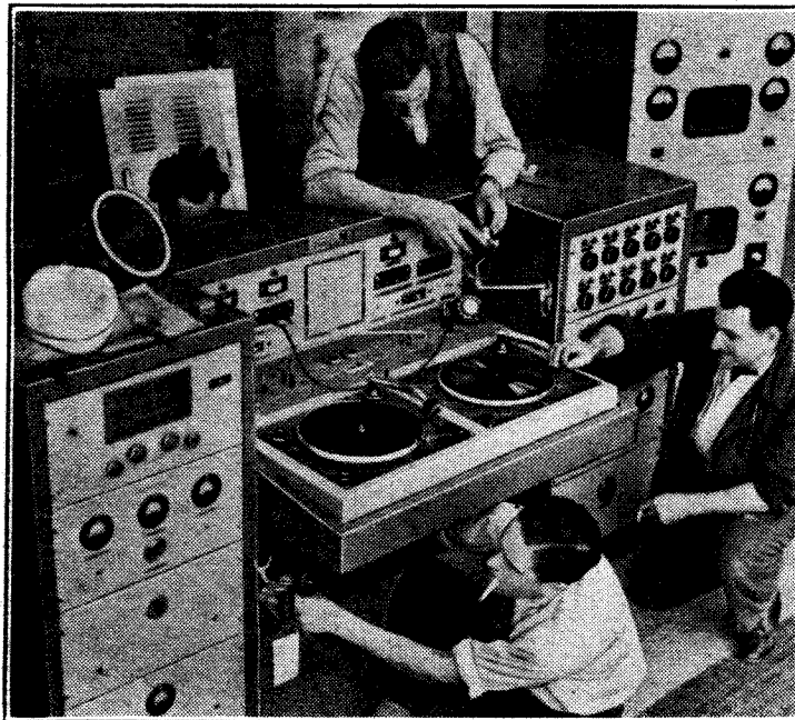
INSTALLING apparatus for the centralised distribution system through which signals for demonstration purposes are fed to the stands at the Salon de la Radio, which opened in Paris on September 1st and continues until next Saturday.
