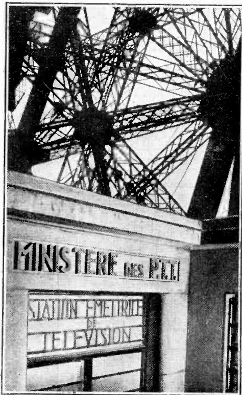
The entrance to the new Paris television station designed and installed by Le Matériel Téléphonique, French licensee of the International Standard Electric Corporation of New York.
