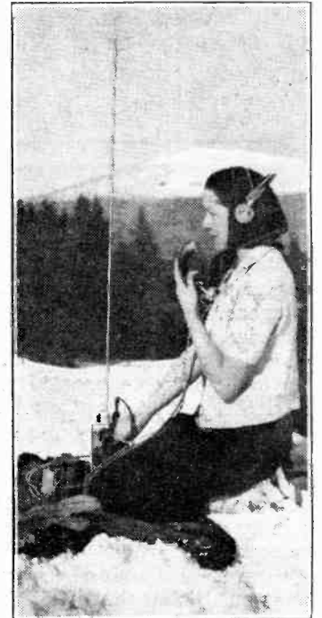
PORTABLE SHORT-WAVE transmitter-receivers were recently tested by Ski-ing Rescue Brigades and the Swiss Army to gauge the effectiveness of wireless in the location and relief of casualties in the Swiss mountains.
