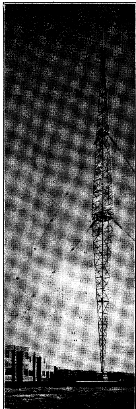
The success of the Lisnagarvy anti-fading aerial has been so marked that it is being adopted for other new transmitters.
