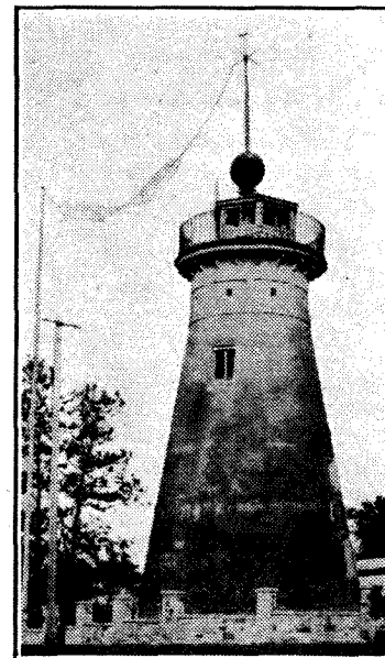
HISTORIC SITE FOR TELEVISION. —Mr. T. M. B. Elliott, of Brisbane, Queensland, has converted this historic convict treadmill tower to a very modern use, as a wireless and television experimental station. The tower is the property of the Government, but has been placed at the disposal of Mr. Elliott for his research work.
