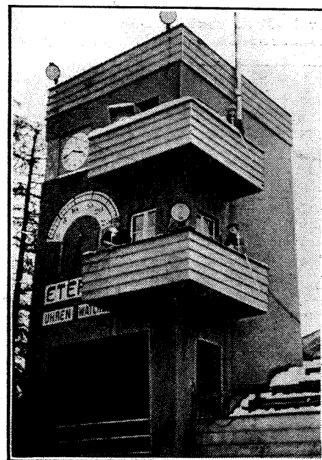
RADIO TOWER at St. Moritz, specially constructed to meet the needs of broadcast commentators on winter sports. Microphone points are fitted for a large number of commentators.
