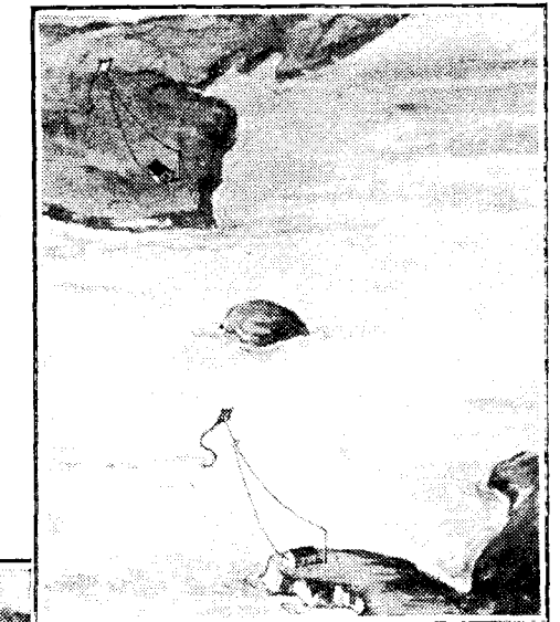
Elevated cylindrical aerials were first used at the Needles station, Isle of Wight. Kite aerials were also experimented with.
