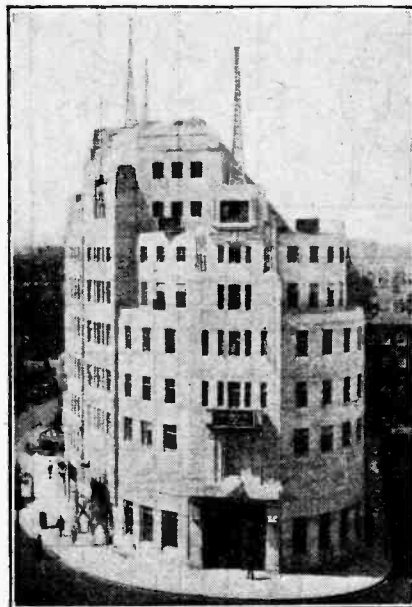
READY FOR LAUNCHING. Like a ship about to be run down the slips, "Broadcasting House" is now externally complete. The interior is still in the crude state, however, and doubts are expressed as to whether the B.B.C. staff can move in before November.
