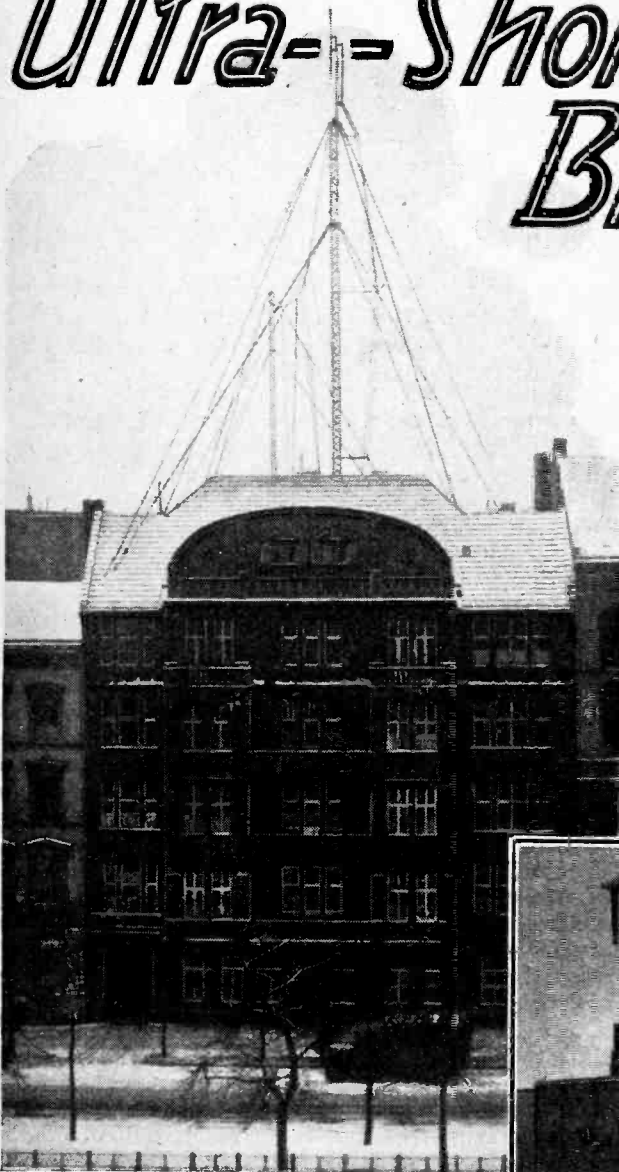
Dipole Aerial of the Telefunken experimental transmitter. Wavelength 7.05 metres.
