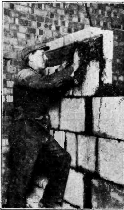
NEW USE FOR SEAWEED. —Among the architectural refinements included in the new "Broadcasting House," Portland Place, are special soundproof studio walls packed with seaweed.
