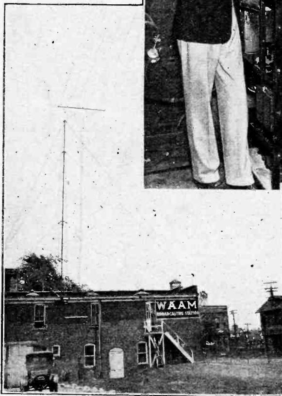
is increasing its power to 500 watts. The new transmitter is seen in the upper photograph, while the lower photograph gives a good impression of the exterior of a typical American low-power broadcasting station. WAAM makes use of a counterpoise, an arrangement which has been found more satisfactory than the original earth system.
