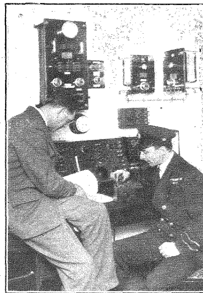
WIRELESS ON NEW LINER. A glimpse into the operating cabin on board the new P. and O. Liner ss. "Ranpura."
