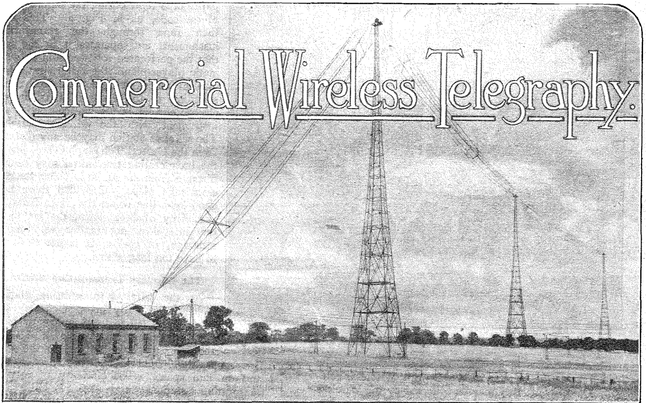
The aerial system and the earth screen at Onga.
