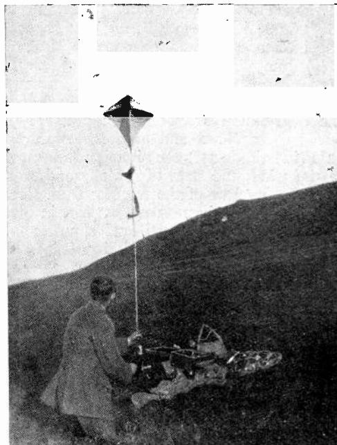
Kite-lifted aerial comprising 600 ft. 20 S.W.G. steel piano wire.
