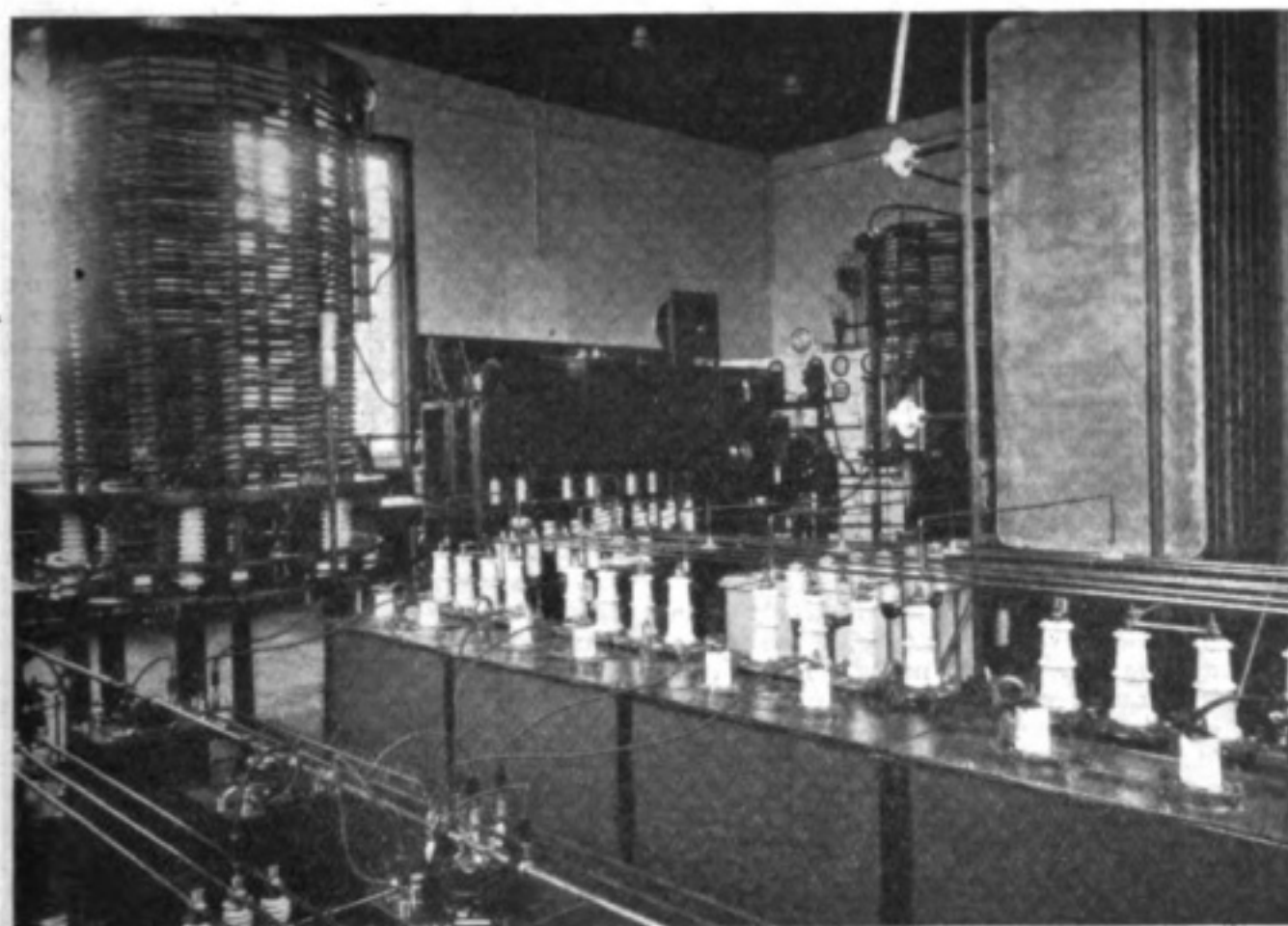
Fig. 9. Another View in the Transmitting Room, showing High-tension Transformers, L.F. Chokes, and on the right the Main Air Condenser.
