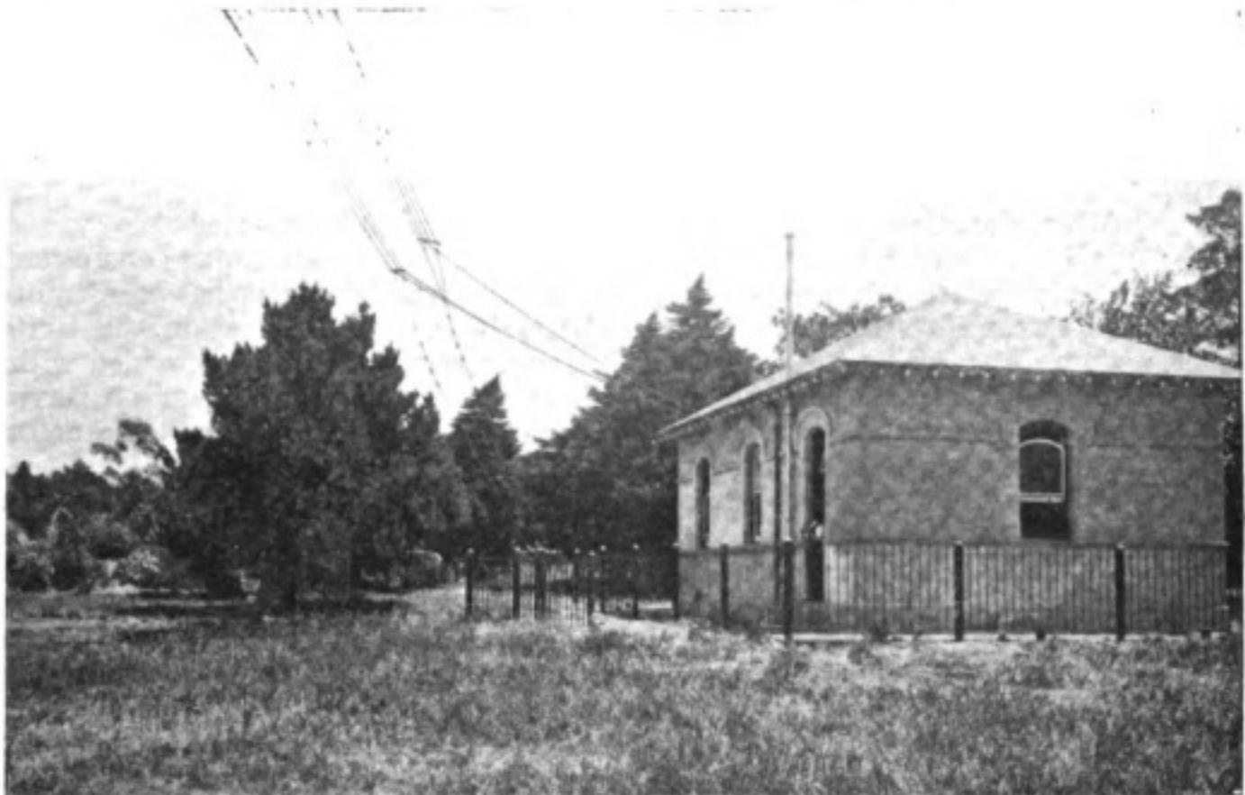
VIEW OF LOWER PORTION OF ANTENNA AT MEL- BOURNE WIRELESS STATION TAKEN FROM THE EAST.
