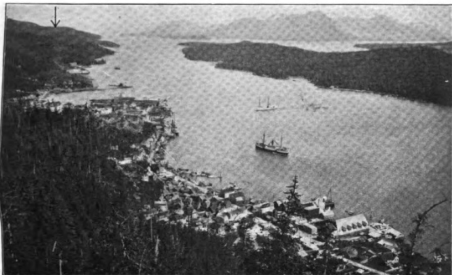
A VIEW OF KETCHIKAN, ALASKA. THE ARROW INDICATES THE CLEARED RIGHT OF WAY OF THE NEW ENGLAND FISH COMPANY'S 3-PHASE 6,600-VOLT TRANSMISSION LINE TO GEORGES INLET, SIX MILES DISTANT.
