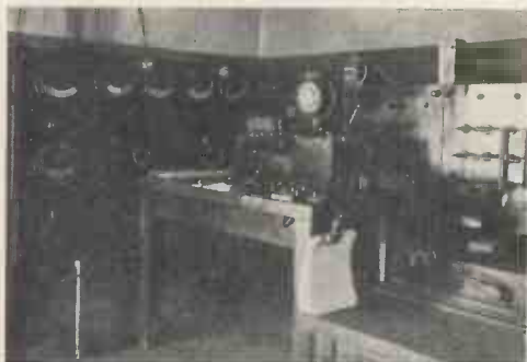
Receiving Instruments and Power Switchboard.
