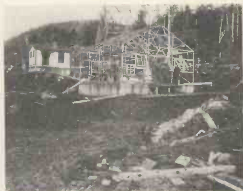
Ketchikan—Operating House completed and Power House under construction.
