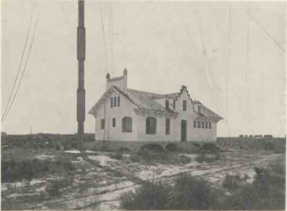
Exterior of Wireless Station Building, Prat de Llobregat, Barcelona.
