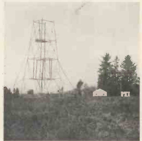
Astoria Station—Two forward Towers under construction.
