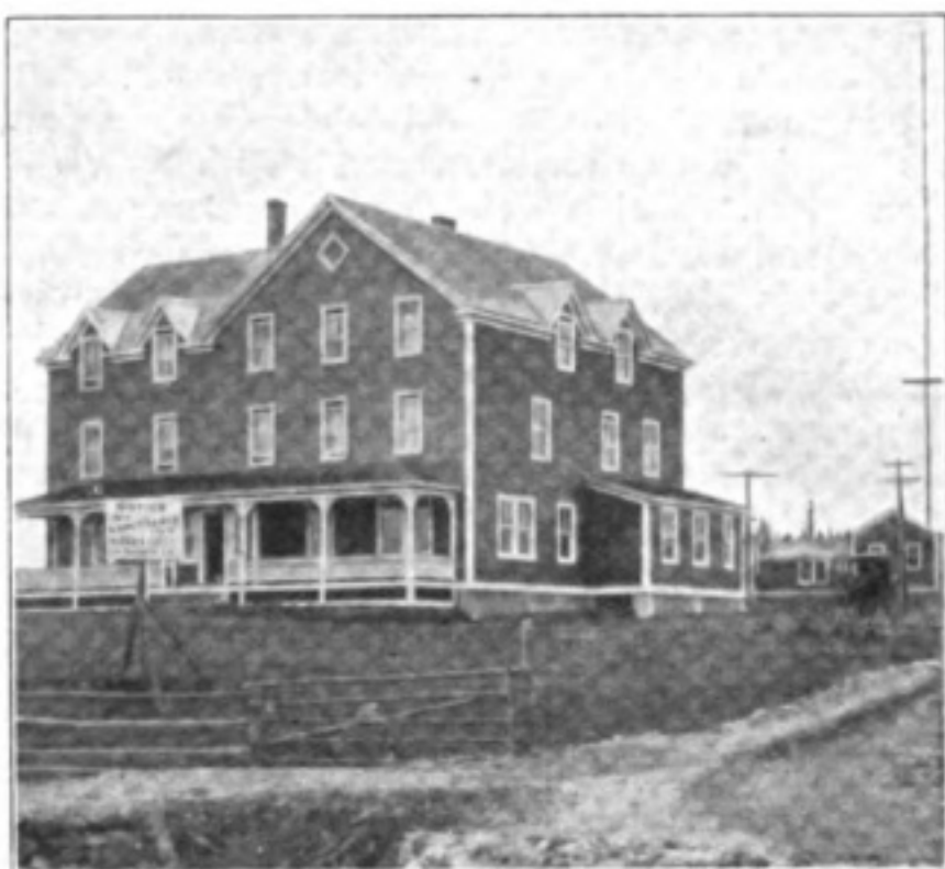
Operators' Quarters at the Wireless Station.
