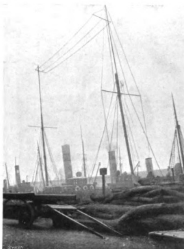
A Hull Fishing Steamer fitted with special masts and Marconi apparatus.
