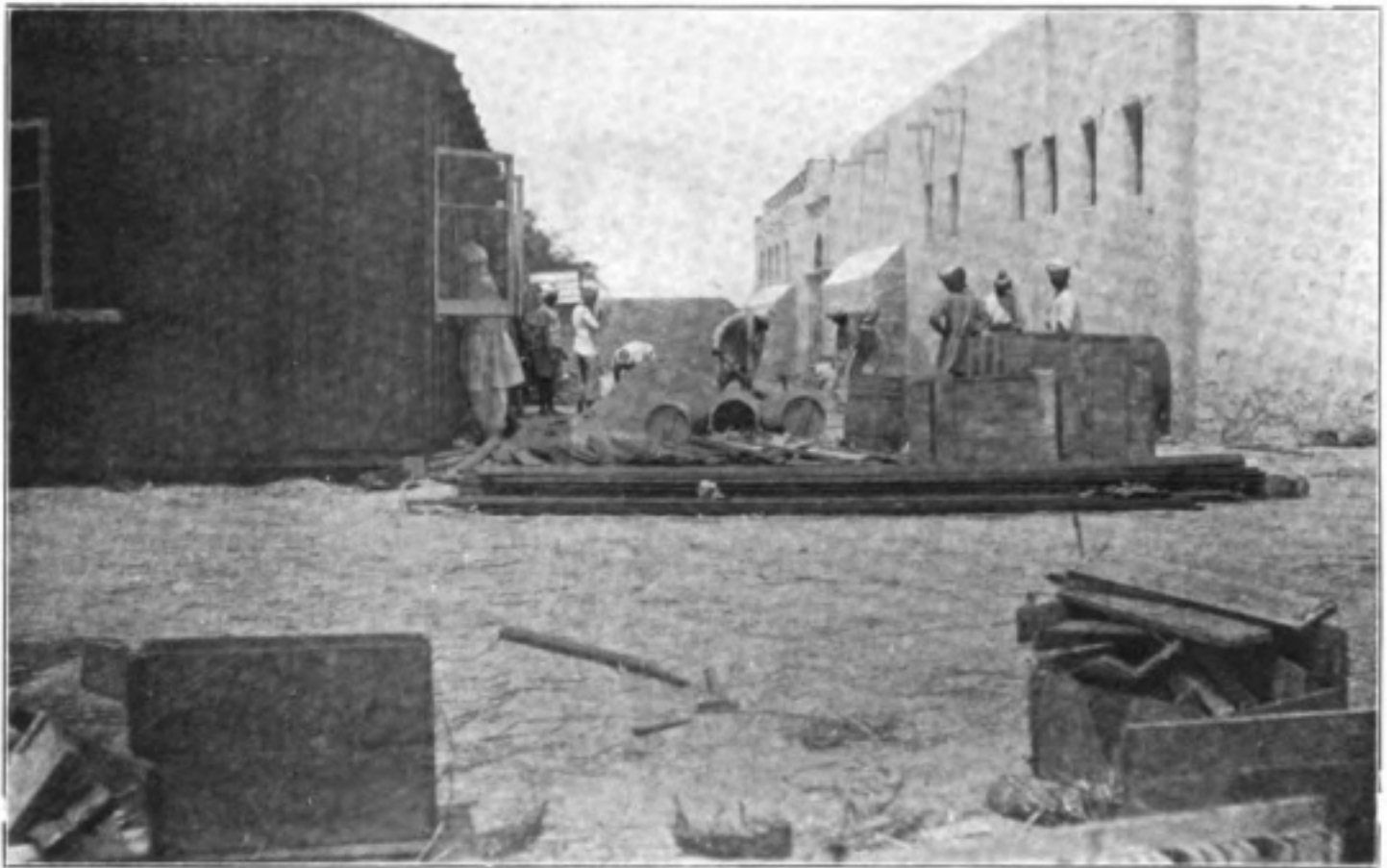
Beluchi soldiers doing concrete work at Berbera
