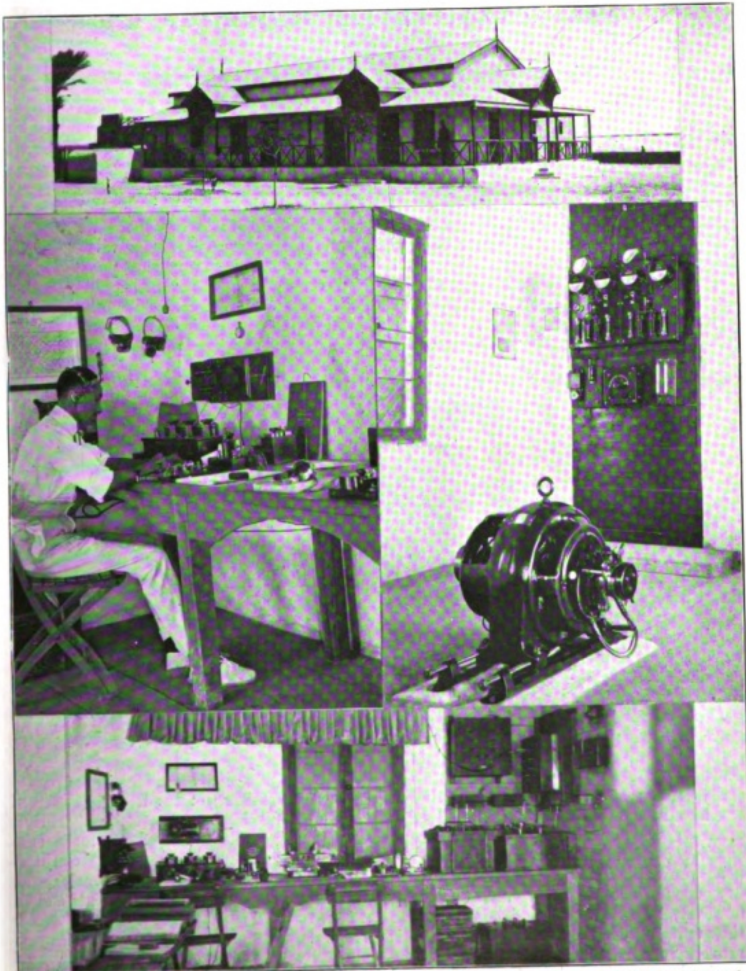
1. The Station. 2. Operator Receiving. 3. Converter and Switchboard 4. Instrument Room.
