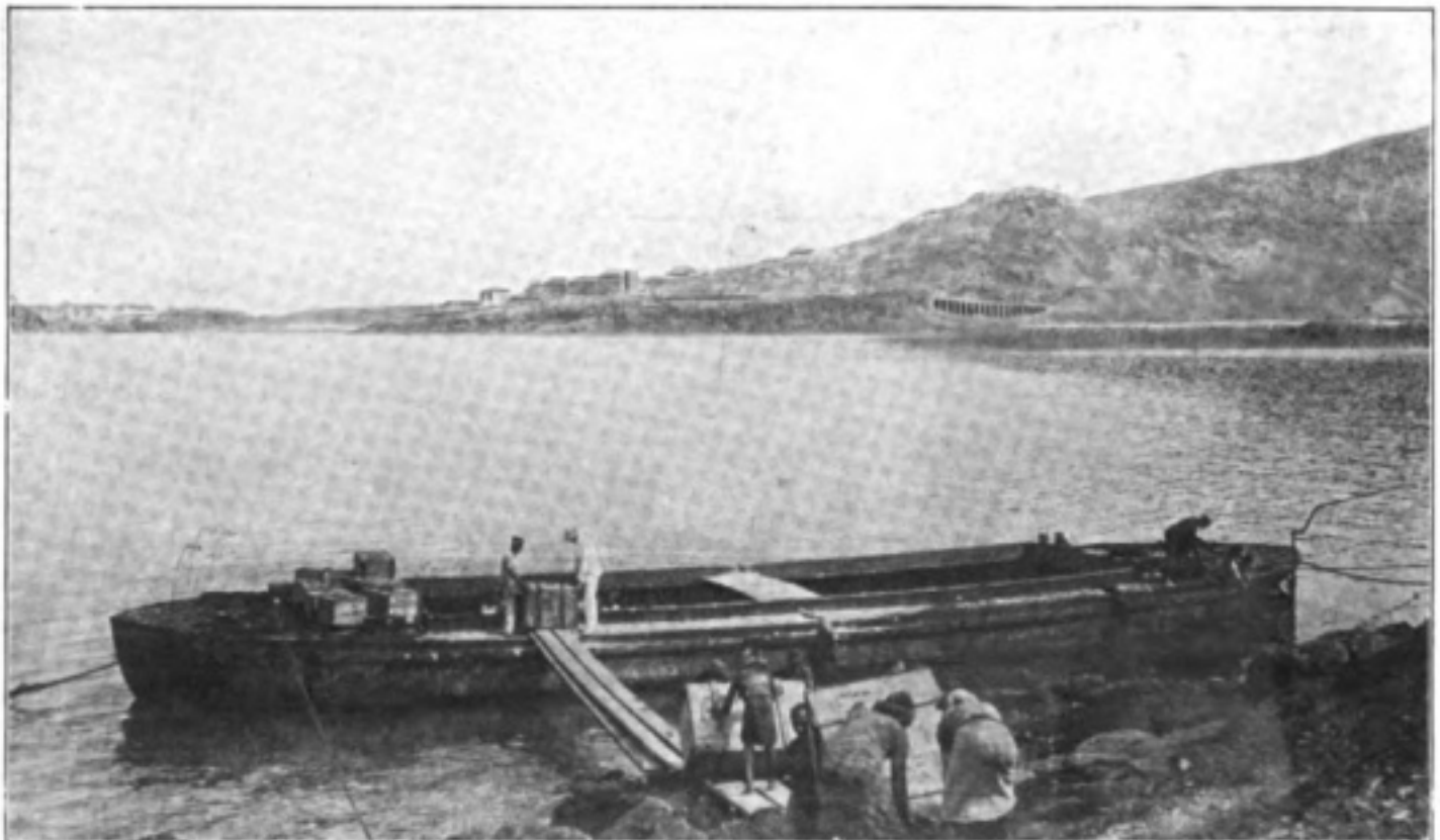
The difficulties of landing materials at Aden. 150 ton lighters must be anchored well out through danger of breaking on the rocks
