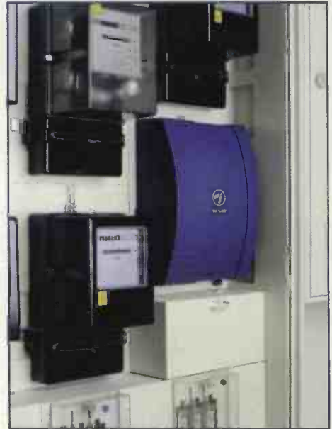
Online box in the electricity meter's cabinet. The box is part of the power utility's infrastructure.
