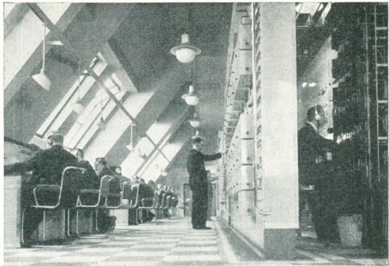
The Empire programmes, like all our home programmes, have to pass from the studios to the main control room at Broadcasting House from where they are sent by landline to the transmitters at Daventry
