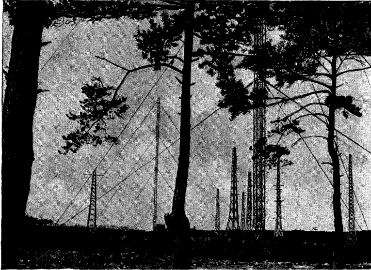
Lusty photo One of the easiest of short-wave stations to log is Zeesen. Here you see the forest of aeriels outside the transmitting house. Remember that a different aerial is used for every wavelength used
