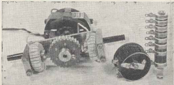
A small television motor fitted with synchronising gear. On the right are two resistances, one variable and the other semi-variable for speed control
