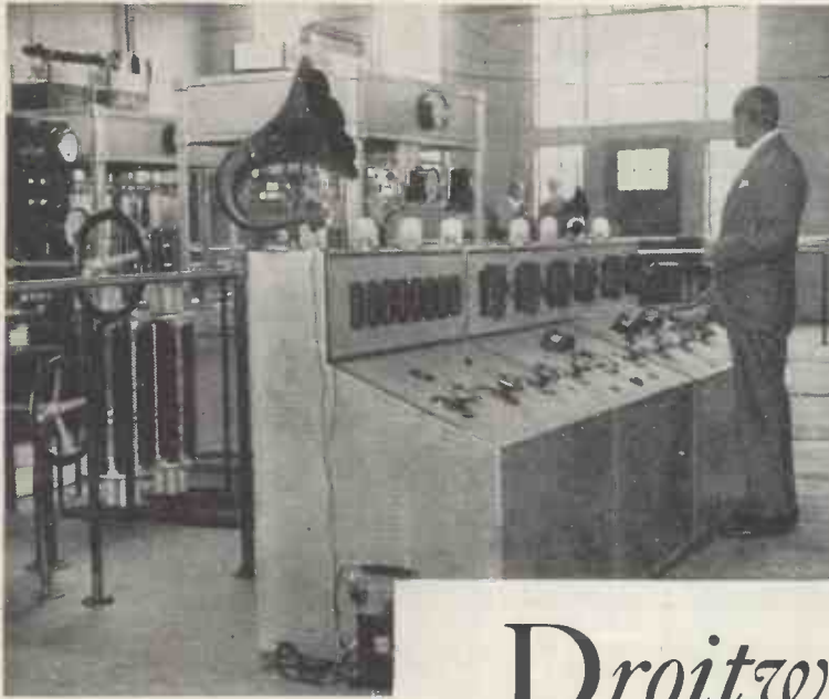
Very soon we shall be hearing the last signals from Daventry National. Here you see the first control panel used in the transmitting hall at Daventry
