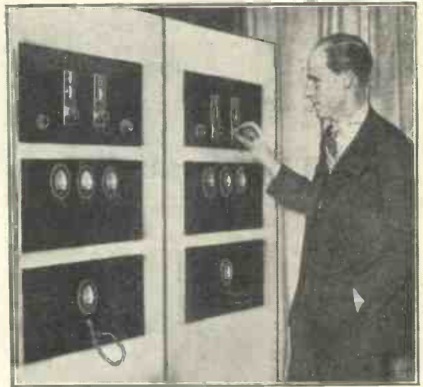
THE RELAY EXCHANGE AT WOOD GREEN The first relay station to distribute alternative programmes to London subscribers. This receiver uses a total of twenty-two valves
