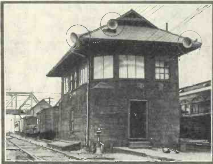
Shunting operations in a Toronto (Canada) passenger coach yard are controlled by a "signalman" through the medium of twenty-five loud-speakers
