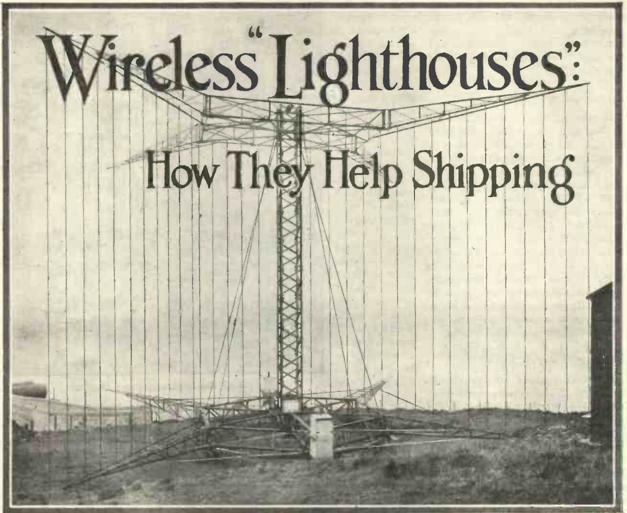
Wireless "Lighthouse" at the Entrance to the Firth of Forth; it was Built by the Marconi Wireless Telegraph Co., Ltd.
