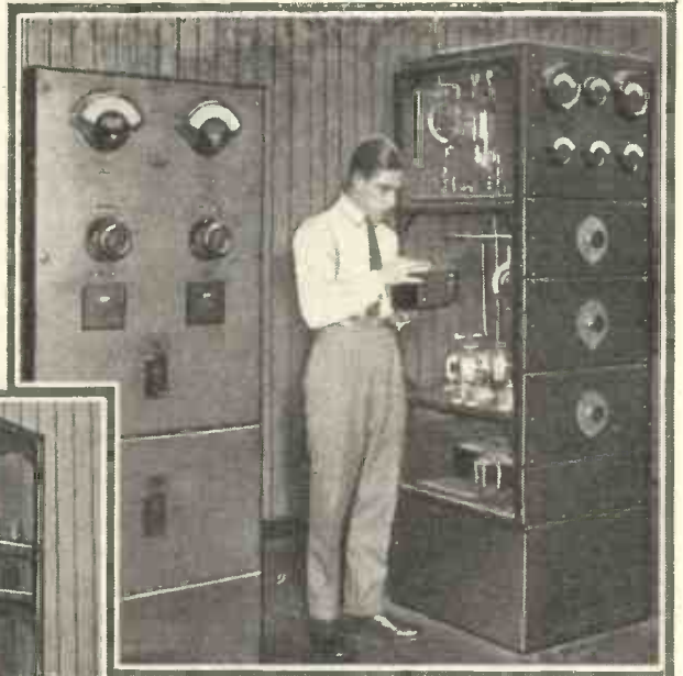
Many English listeners are familiar with San Sebastian, EAJ8. These photographs show the engineer attending to the transmitting gear; on the left he is adjusting the aerial tuning and above he is measuring the wavelength before starting to transmit a programme.
