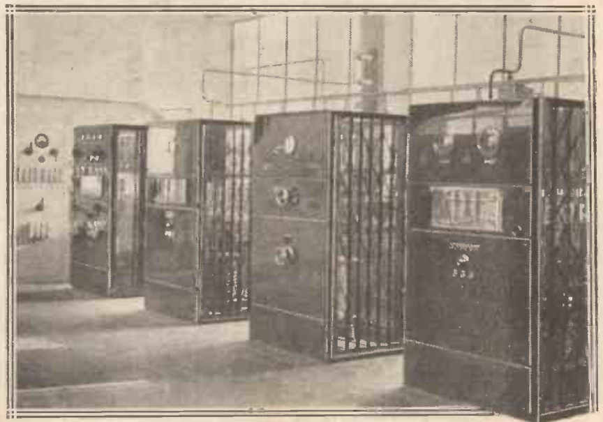
Here we see the transmitting panels at Radio-Suisse Romande (Sottens), the well-known Swiss broadcasting station which works on a wavelength of 403 metres. Using a power of 25 kw., Sottens is separated by only 9 kilocycles from the Midland Regional's wavelength.
