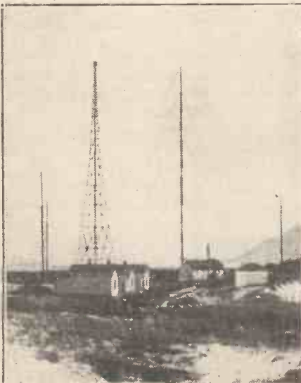
Here you see the principal South African radio station. It is situated at Slung Kop, about 50 miles from Cape Town, and was recently fitted with new aerial towers.
