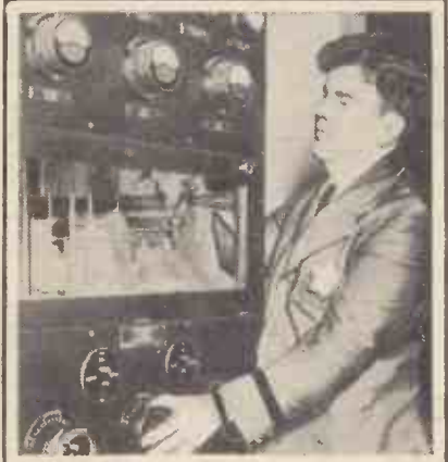
The new radio transmitter at the Chicago Central police station. The transmitter is used for communicating with Flying Squad vans.
