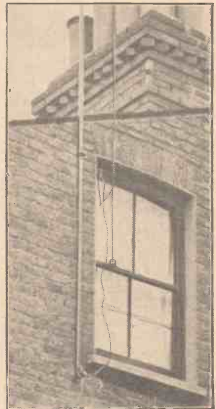
Fig. 2.—Showing how the mast was securely fixed in position and the down lead arranged.
